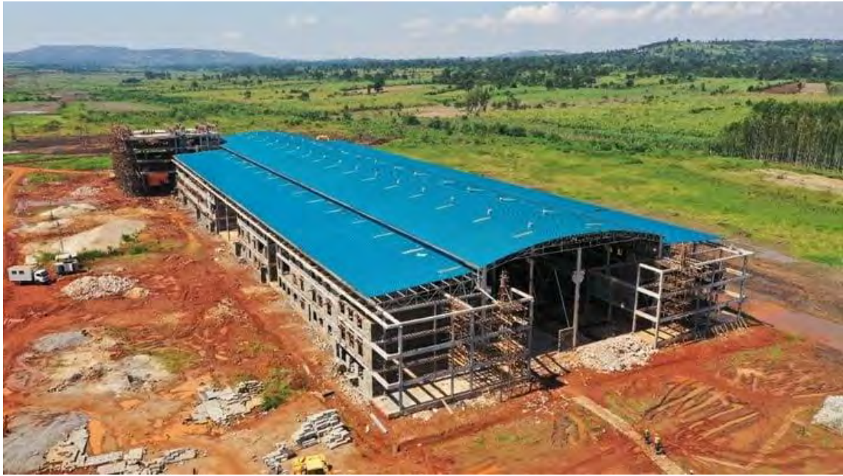
Figure 3.15: Status of Construction of Phase I Kiira Vehicle Plant Facilities September 2020
