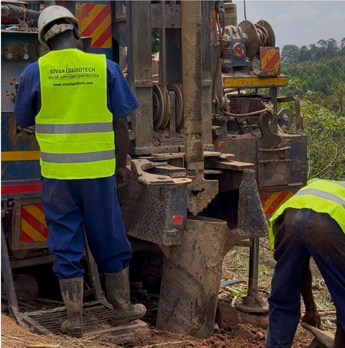
Figure 10-4 Drilling bit and 8-inch casing
