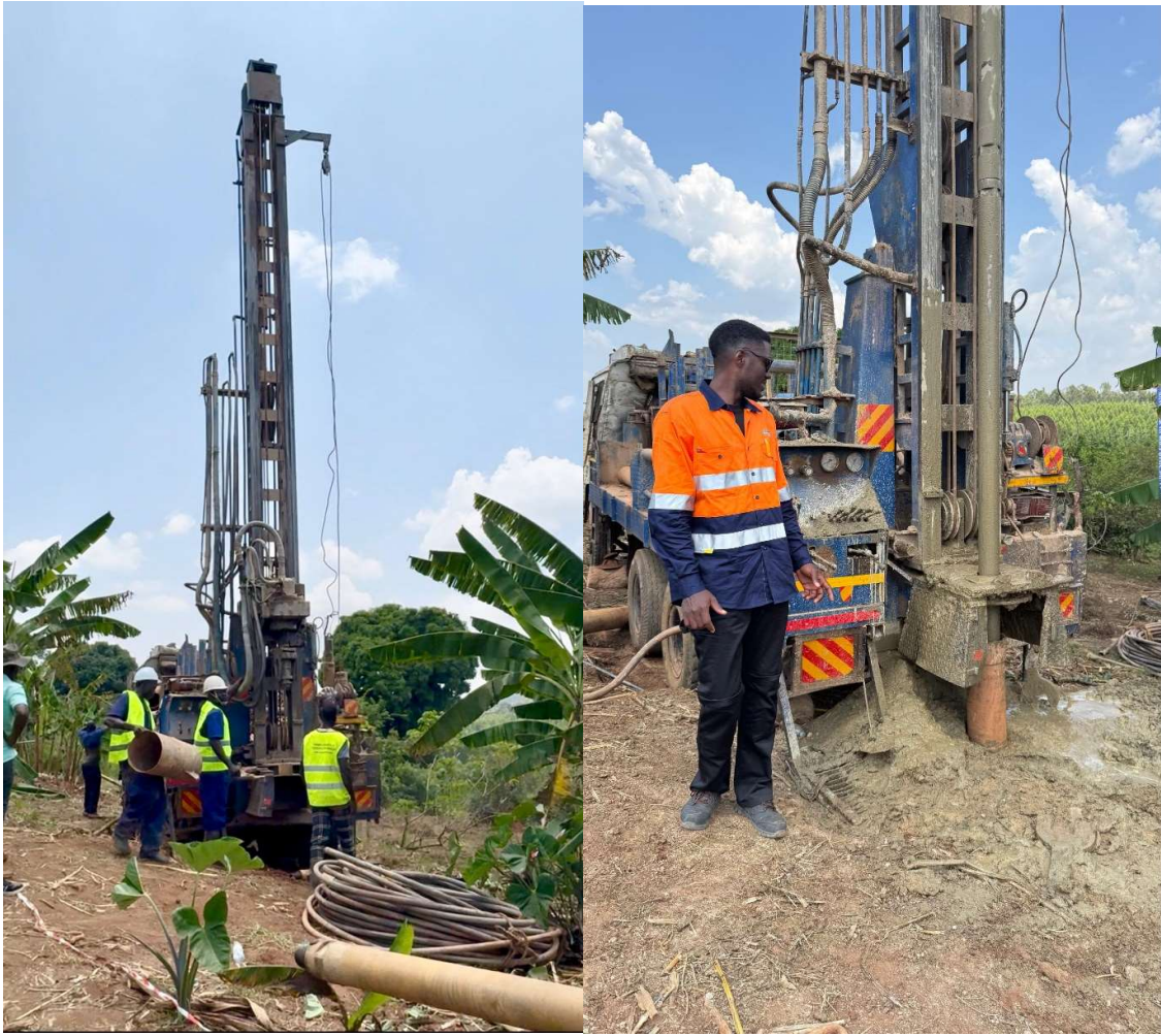
Figure 10-3 installation of casing
