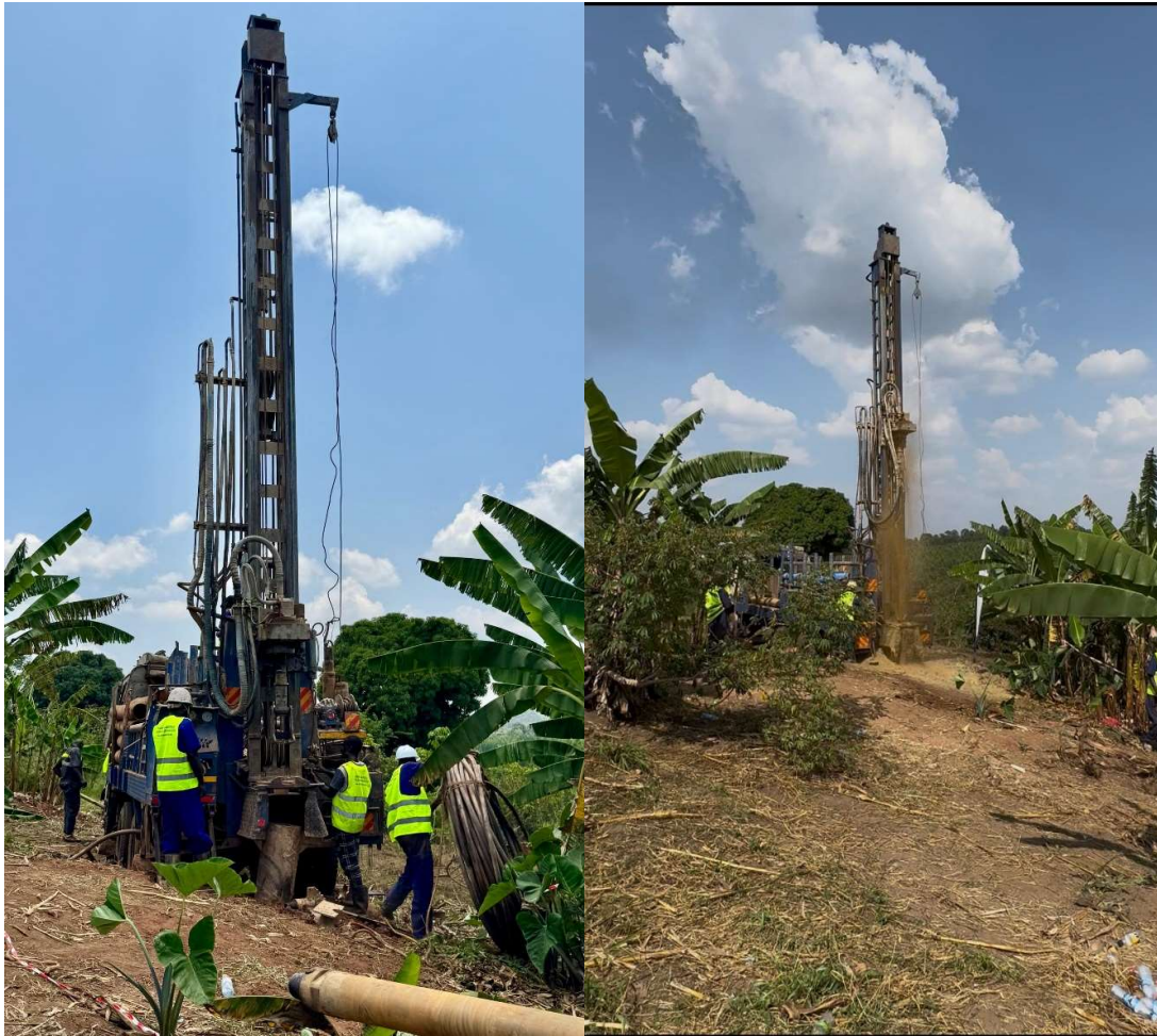
Figure 3-1 Setting up a drilling rig
